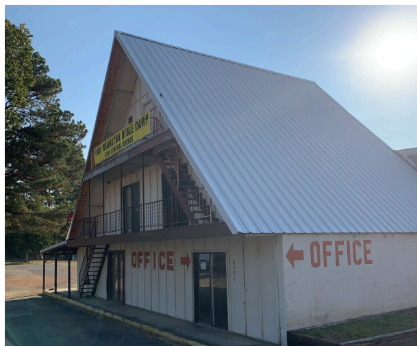
New roof on A-frame after hail damage
